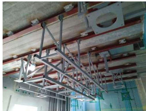
Fig. 353 Auxiliar structure for hanging ceiling equipment at ÖH.
