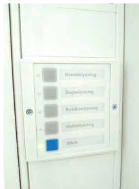
Fig. 261 Light switch for different options: day, evening, night and exploration. ULKÖ.
