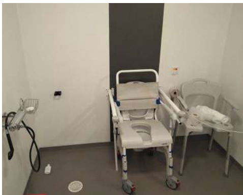
Fig. 239 Patient's bathroom with flat shower and contrasting colours. SKU.
