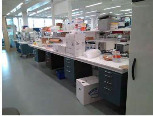
Fig. 114 Laboratory room. Drawers hang from the table to facilitate floor cleaning. KI NKS.
