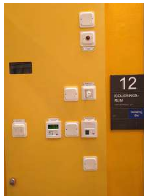
Fig. 82 Air conditioning switches for positive or negative pressure, regulable both in the anteroom and the bedroom. Display to show the type of patient: contagious or immunocompromised. SKU.
