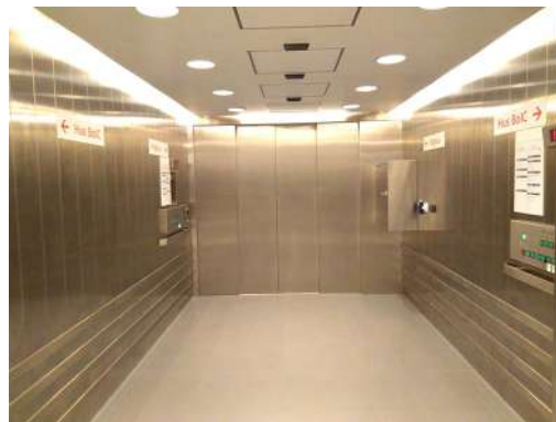
Fig. 51 Internal lift for bed-ridden patients with a specific gases box for patient provision in case of lift failure. SAHLH.
