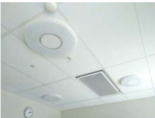
Fig. 260 Ceiling equipment for artificial lighting, air conditioning and fire detection. ULKÖ.
