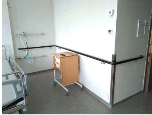
Fig. 256 Handrail from bed to toilet. ULKÖ.
