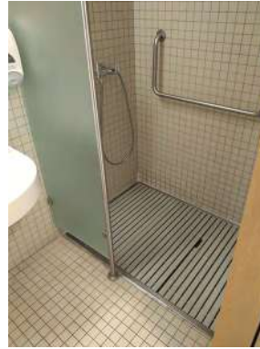
Fig. 303 Flushed shower in the patient's bathroom. MGM.
