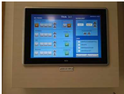
Fig. 142 Environmental conditions control for the patient room. SAHLH.
