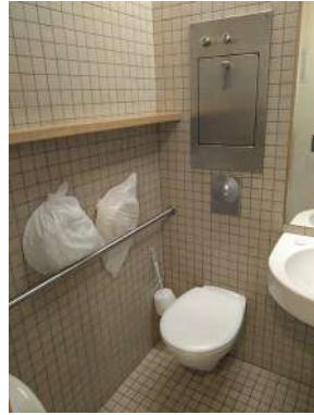
Fig. 302 Patient's bathroom with small tiles. Joints coordinated in the three dimensions. MGM.
