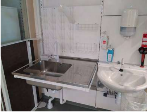
Fig. 113 Ante room for staff hygiene preparation before entering the laboratory. Flexible fixings for easy redesign. KI NKS.
