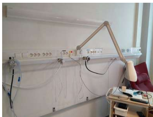
Fig. 235 Detail of headboard equipment with rail to move gas tubes. SKU.
